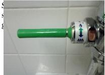
have a flow rate of approximately 2.2 gallons per minute. Replacing these se labeled faucets can reduce the flow from the sink to approximately 1.5 ount for a 30% reduction in water consumption.
